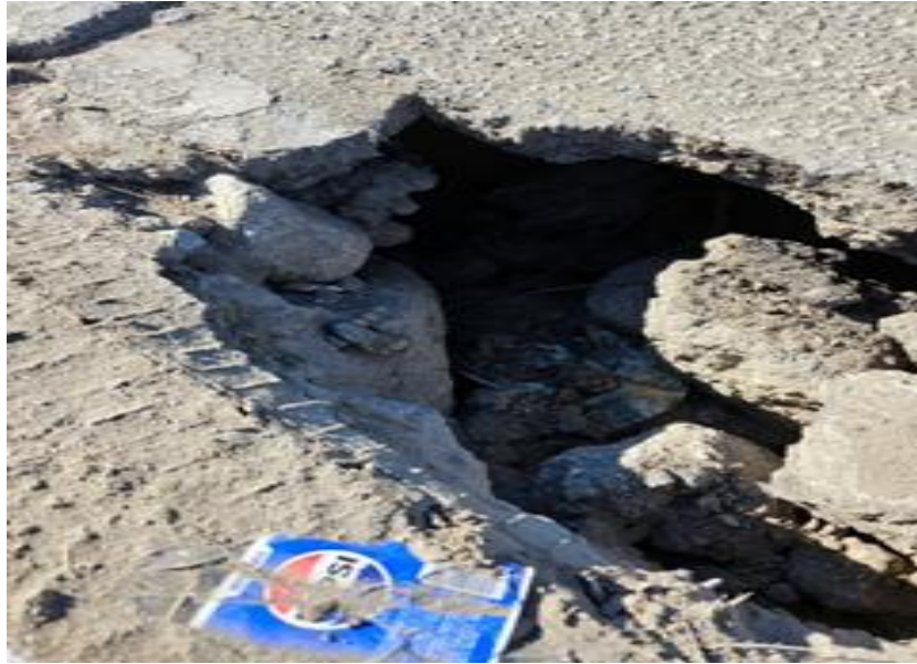
C. Photo 4 – East side of Martinez Road of Culvert.
