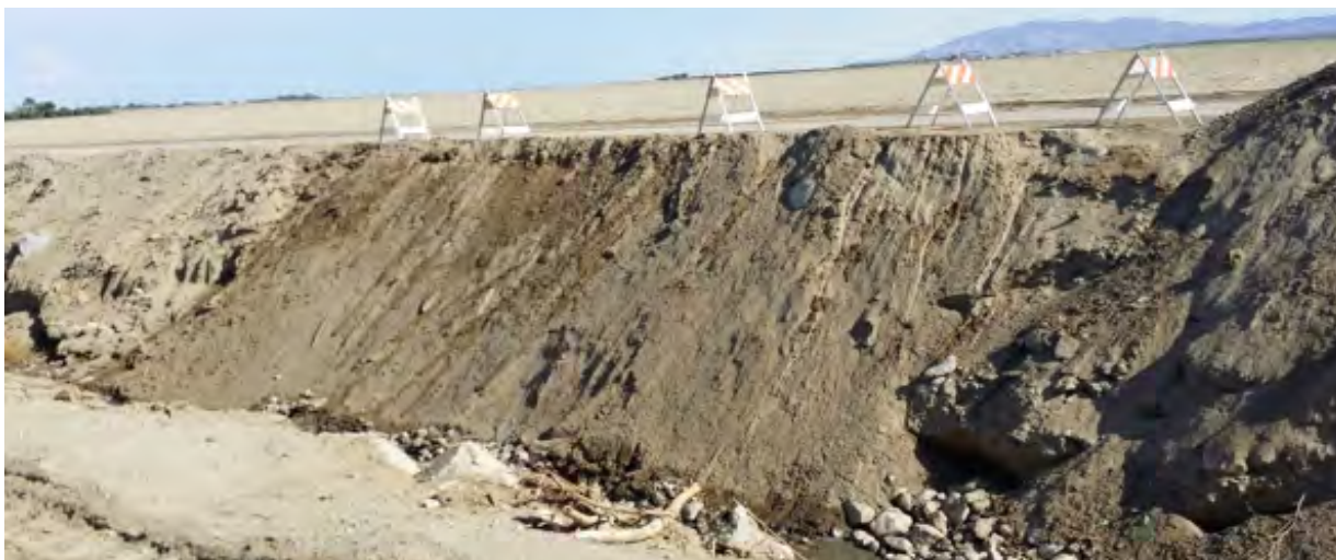
Figure 19. The Repaired Embankment.
